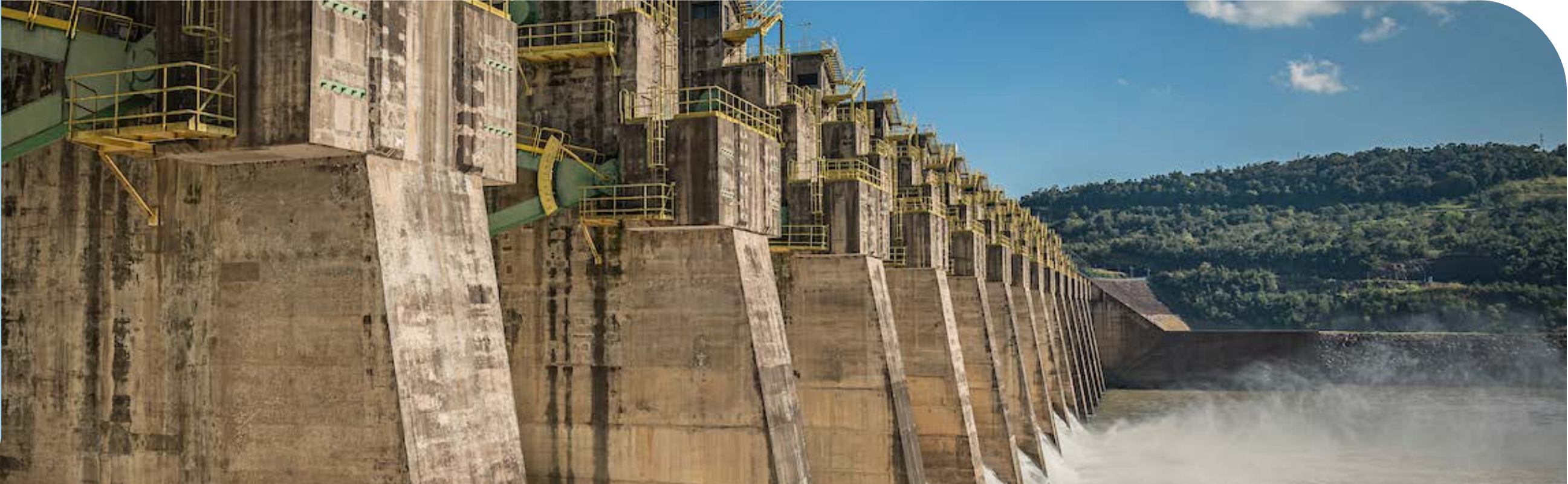
Foz do Chapecó HPP in Santa Catarina (SC)
