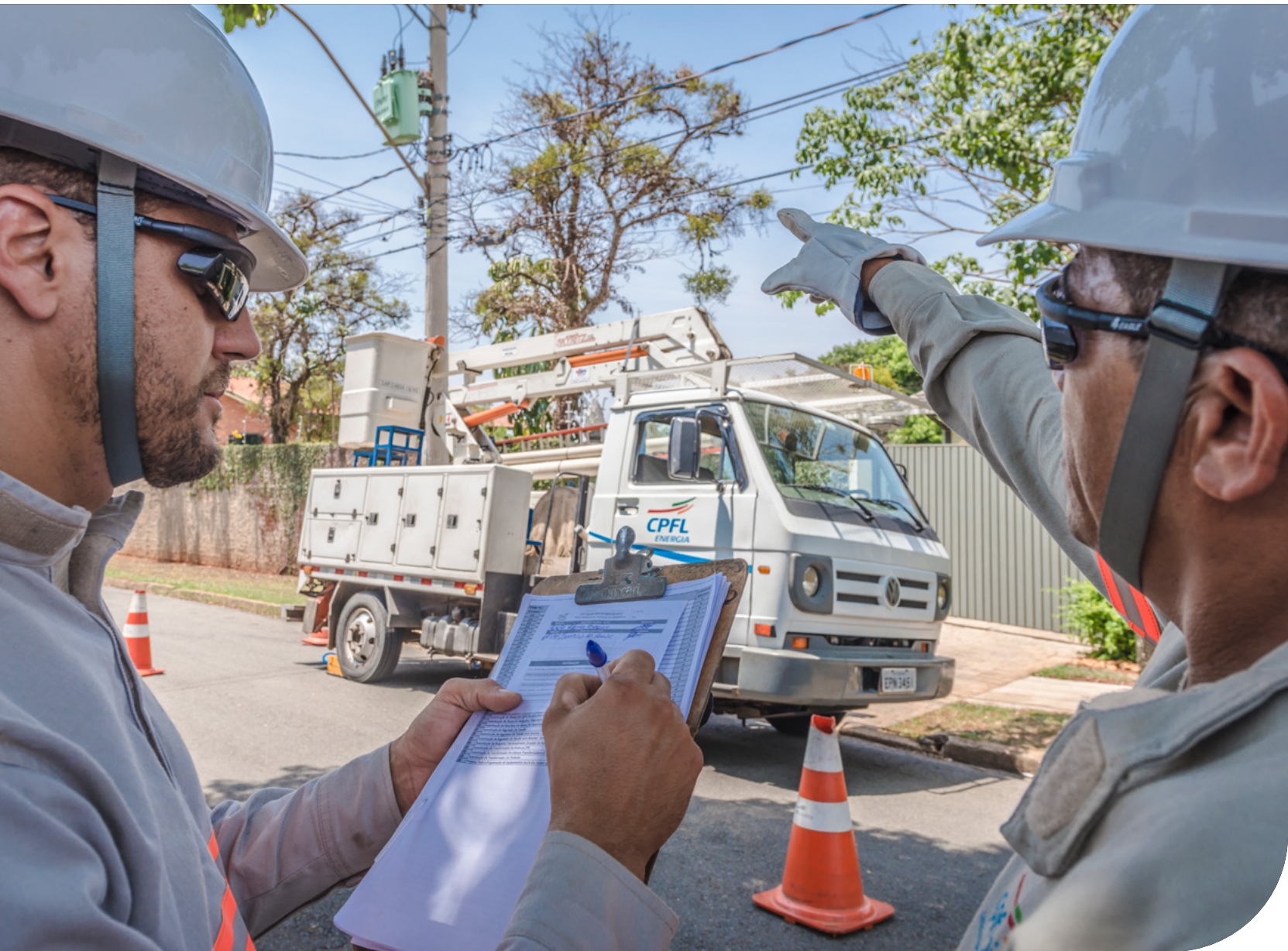
Risk assessment before carrying out work in Campinas (SP).
