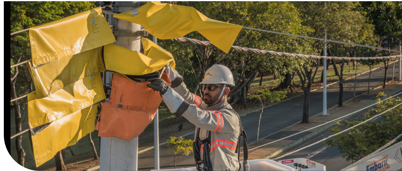
CPFL Piratininga network maintenance (SP).
